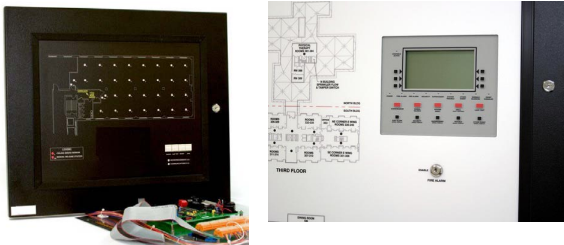
Examples of Annunciator Panel
